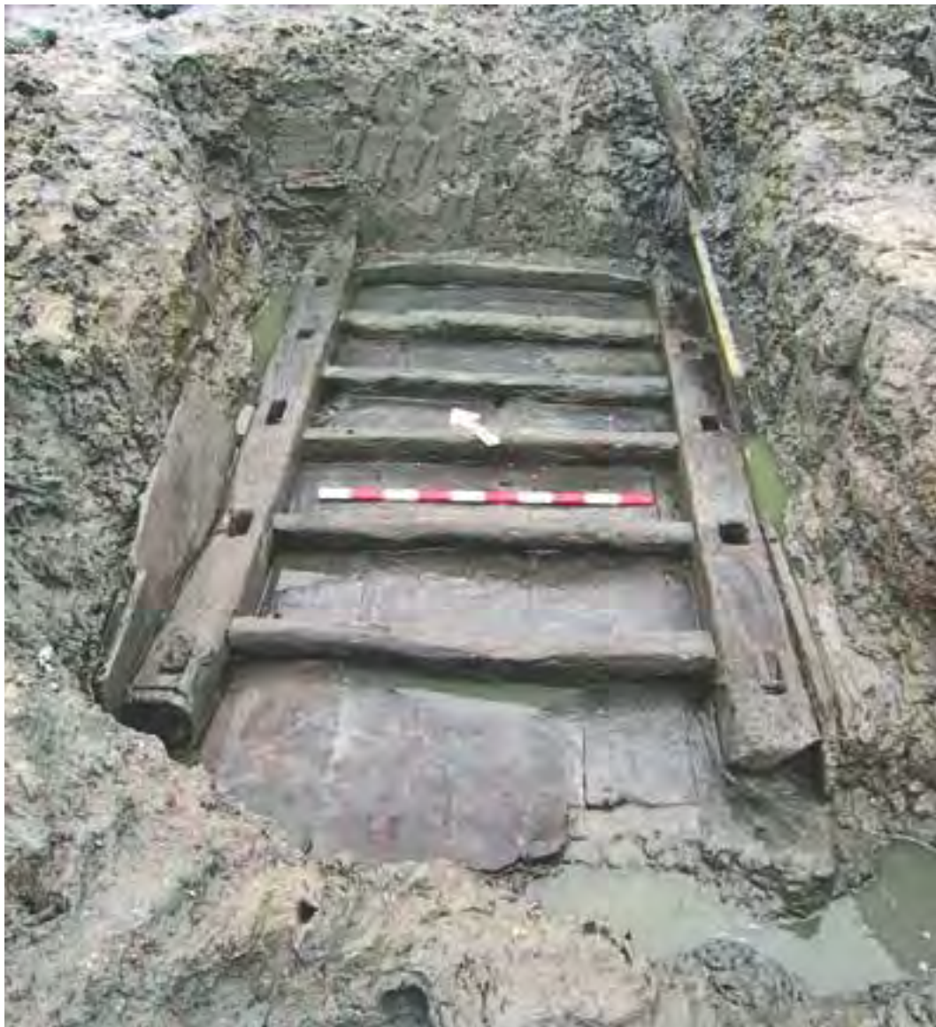
Wooden tidal outlet gate from late medieval times of Seriem, Backbarrier Tidal Flats of Langeoog (Niederhöfer 2010).
